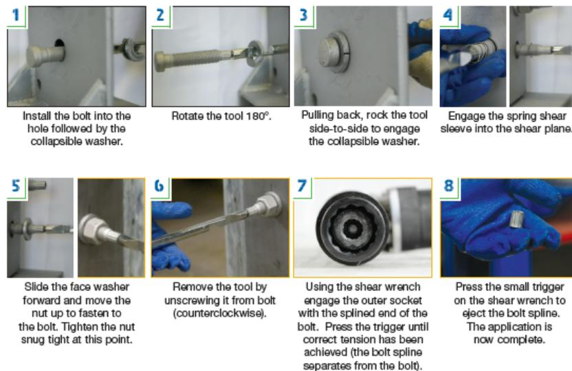
1 Install the bolt into the hole followed by the collapsible washer.
